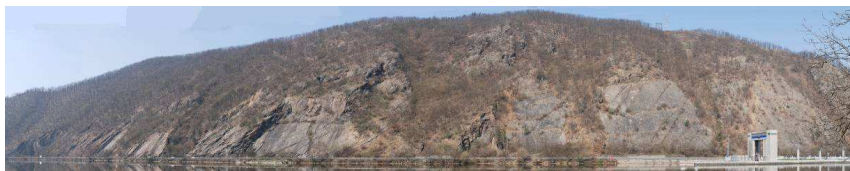
Figure 2. View on the section with highest risk - Vrané nad Vltavou section
