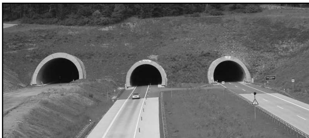
Fig. 2 Behringen Tunnel in Germany
