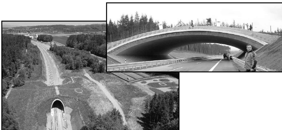
Fig. 5: Green bridges on the motorway A71 in Germany
