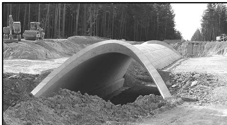
Fig. 3 Green bridge on the motorway A71 in Germany under construction
